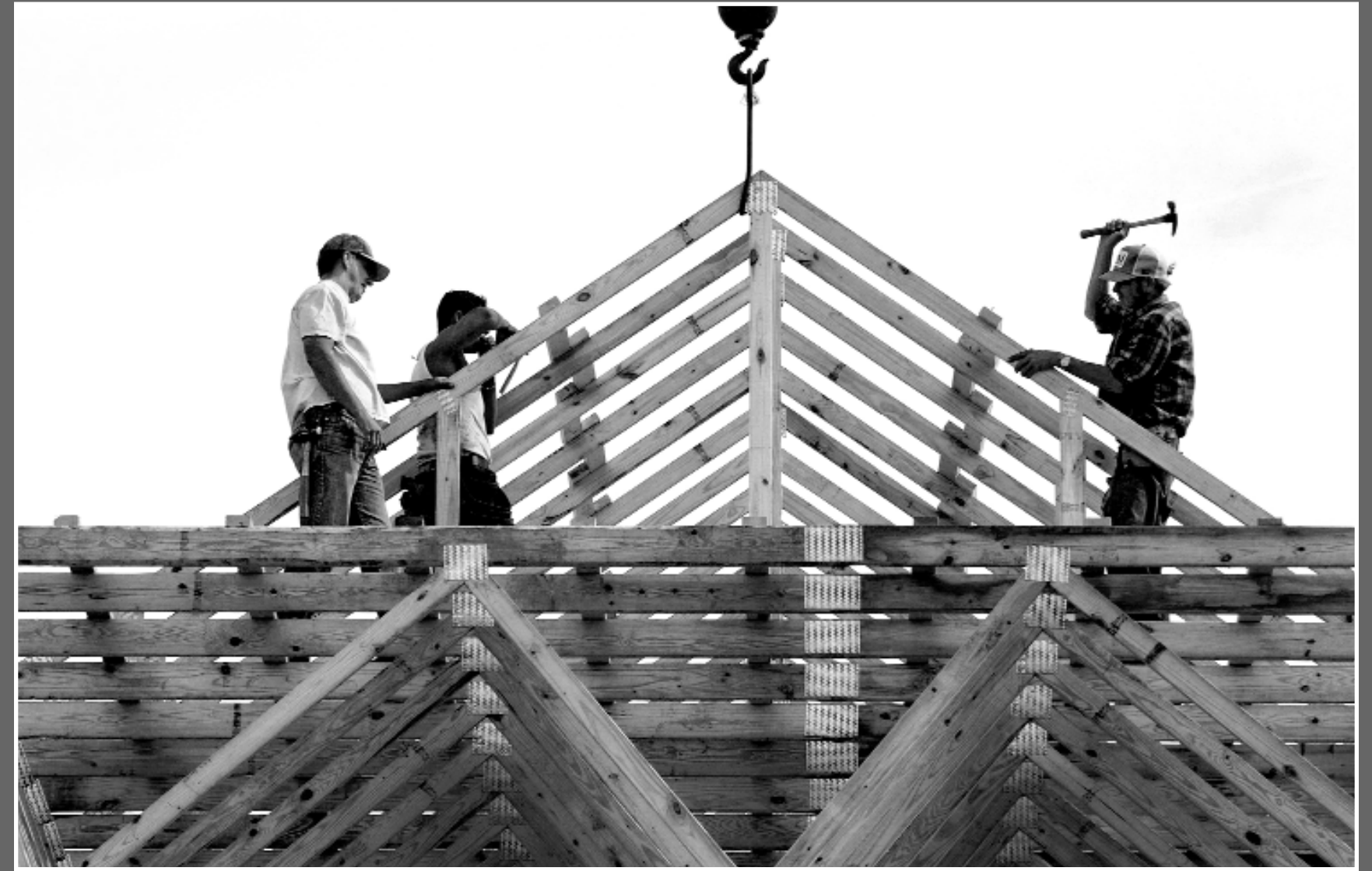
Framers from J.L. Hutchins Designers and Builders attach spacers to roof trusses at the First Christian Church in Bardstown.
