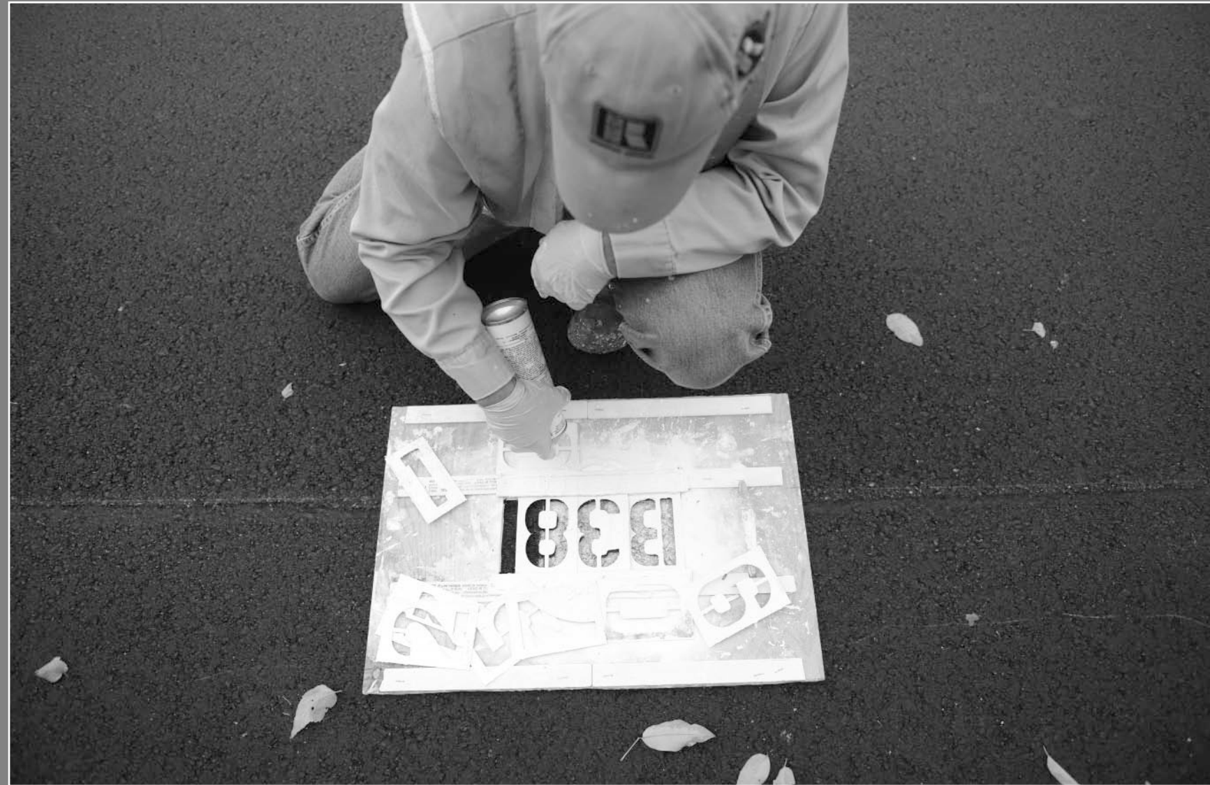
Tim Lashbrook, traffic control worker for the city of Henderson Public Works department, spray-paints parking lane numbers on the freshly paved Main Street.
