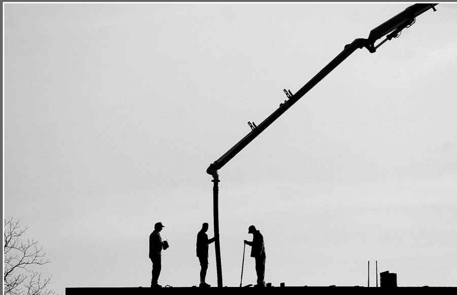
Three men use a boom pump to pour concrete foundations on a farm off Highway 151 in Lawrenceburg.
