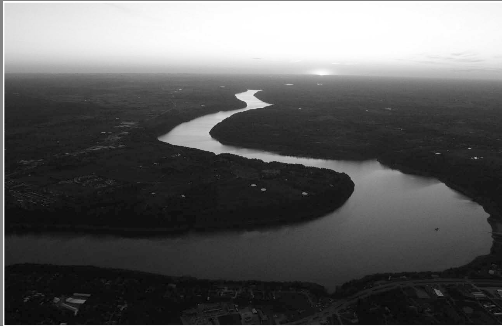
The sun sets beyond Lake Cumberland in Pulaski County. The lake is about 50 feet below its normal level because of a crack in the Wolf Creek dam.
