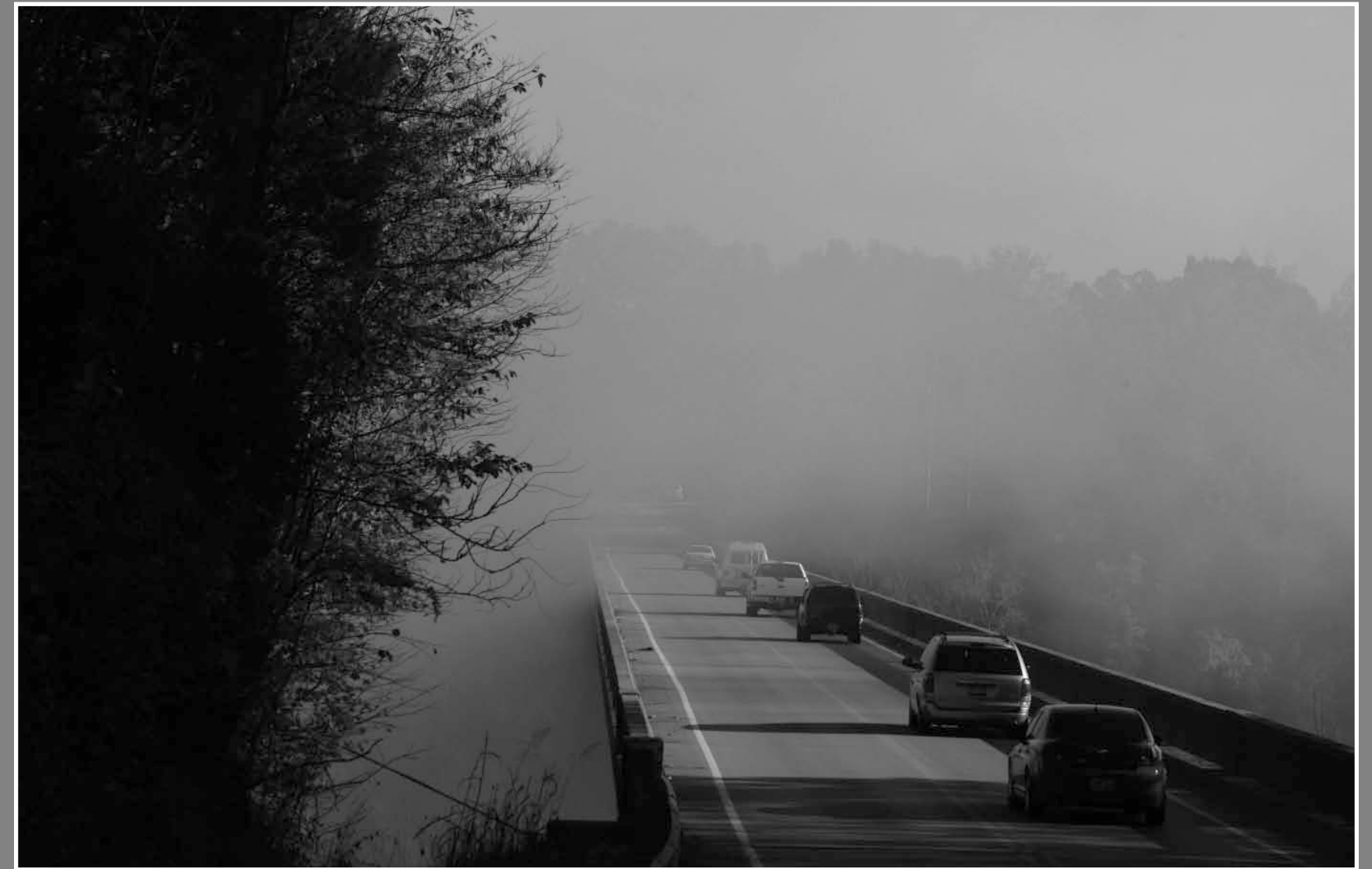
Vehicles drive over a bridge on Highway 80 that spans the Fishing Creek tributary.
