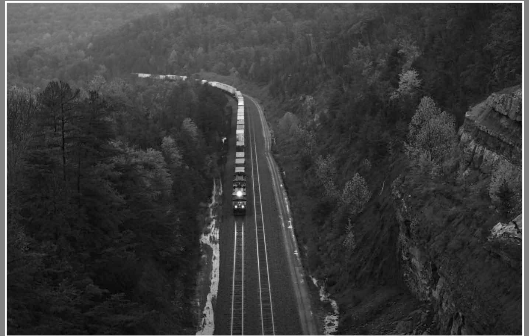
The Norfolk Southern Corp. railroad "Rathole" double-track mainline goes through Burnside, south of Somerset. The track runs along the former Cincinnati, New Orleans and Texas Pacific Railroad right-of-way. The line handles dozens of coal and mixed-freight trains per day. It got the name "Rathole" because it passes through multiple stone-cut tunnels between Burnside and Harriman Junction, Tenn.
