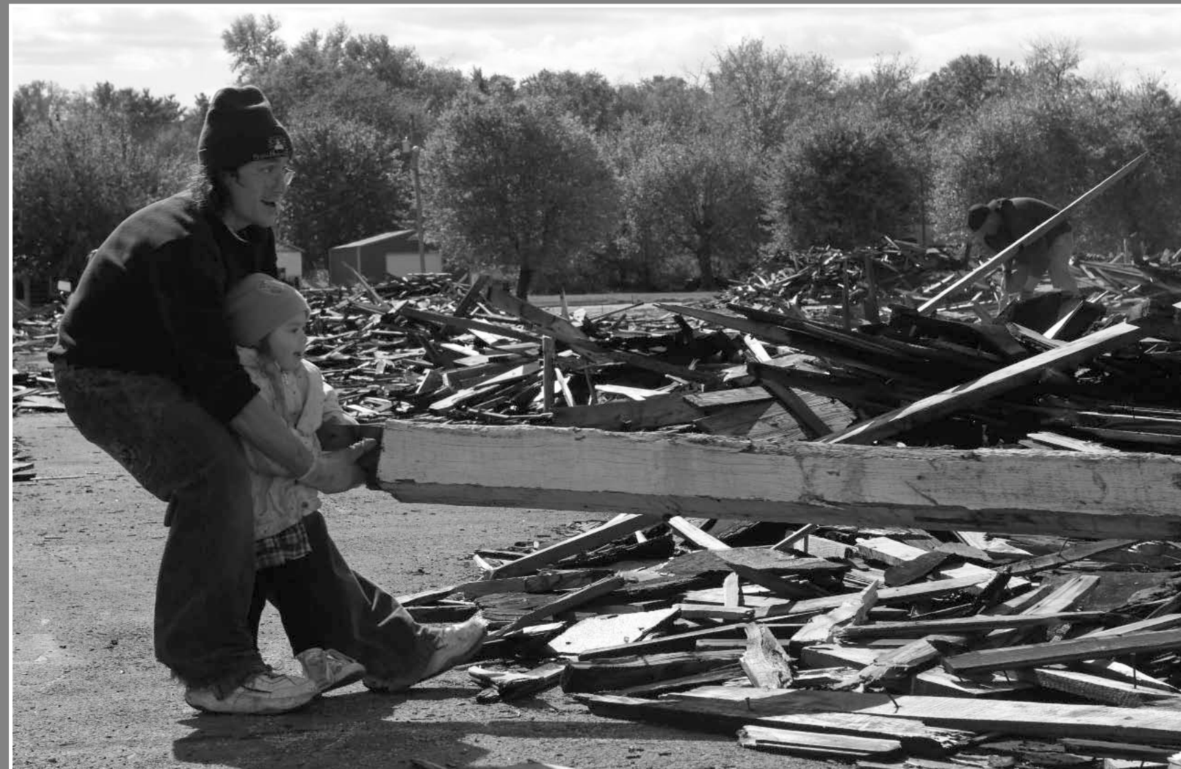
Nick Palmer and his daughter, Inasent Palmer, pull a large timber from the rubble of a demolished tobacco warehouse across from the Pulaski County Board of Education in Somerset.
